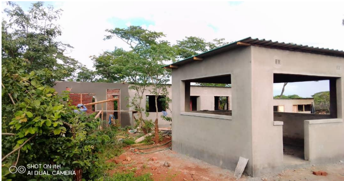
Side view of the kitchen
