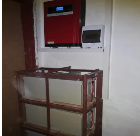
Solar panels, 5KVA inverter and batteries. This was before painting commenced.
